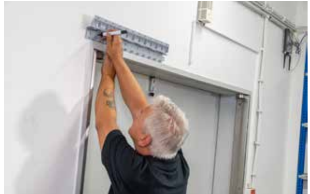
2. Mark and drill the fixing holes
